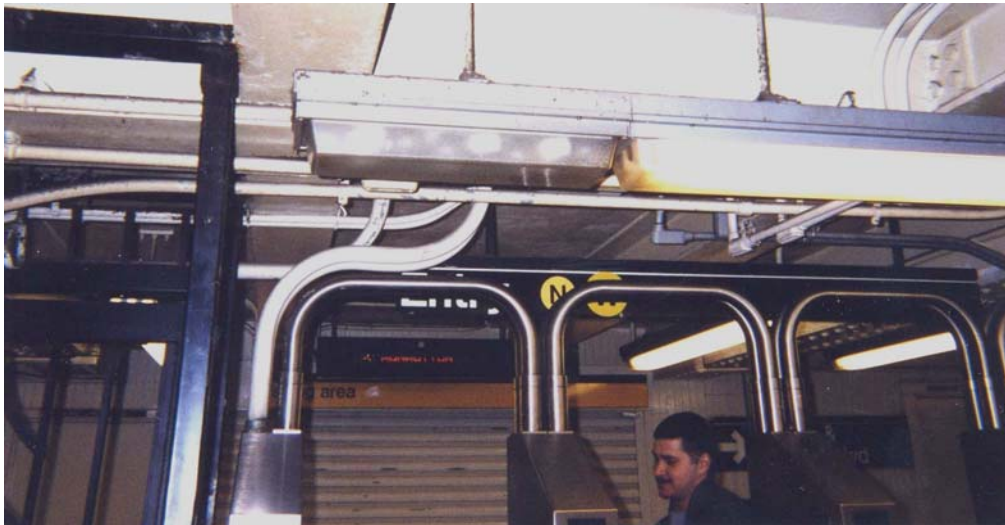
36 th Avenue station, Queens (N/W). The turnstile sign is blocked by the High Entrance Exit Turnstile, light fixtures, and pipes.
