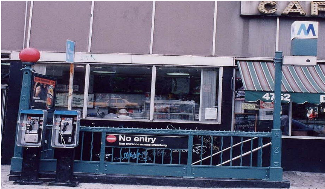
Dyckman Street station, Manhattan (A). An exit-only stairway with two globes-- one green, one red.
