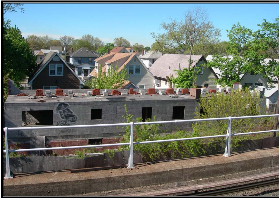
South Side of Laurelton Station
