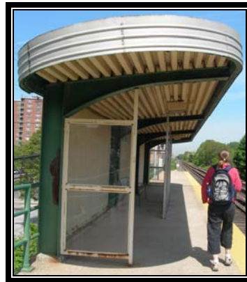
Shelter at Locust Manor
