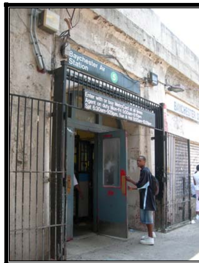
Baychester Subway Station
