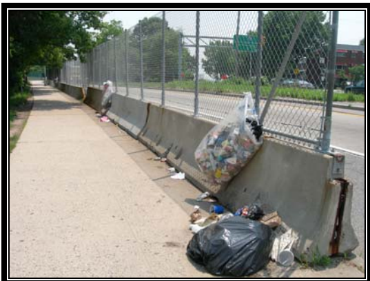
Walkway from Co-Op City to Baychester Subway Station
