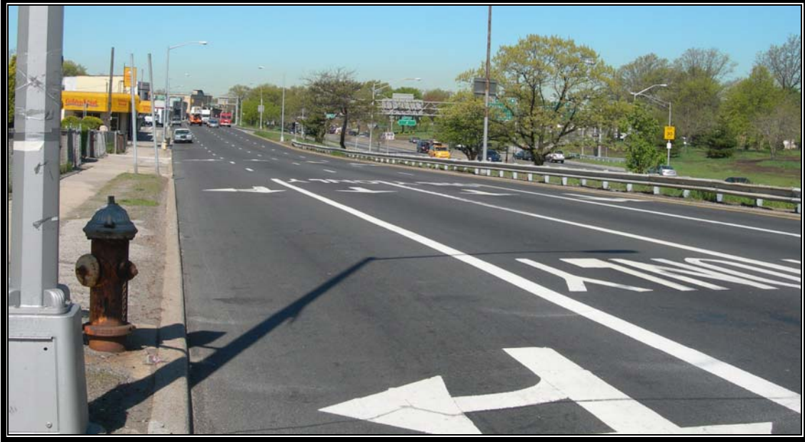
South Conduit Avenue Looking West from 225 th Street
