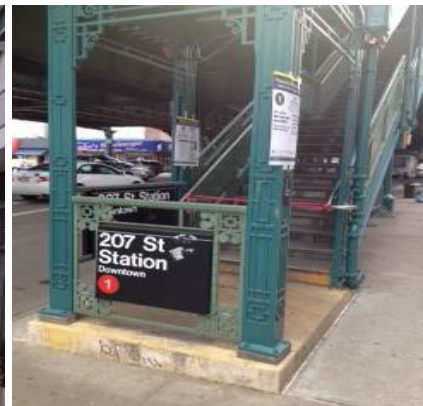
Station entrance signage with red tape
