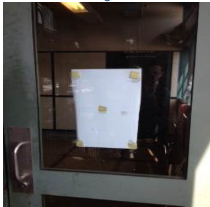
Inaccessible sign location
