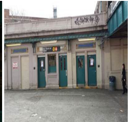
Signage at station entrance
